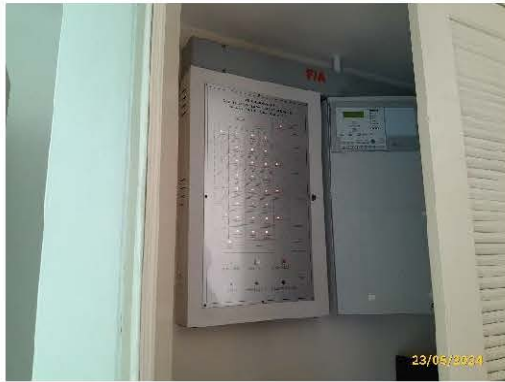
Fire Alarm Control Panel
